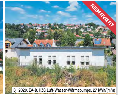
Bj. 2020, EA-B, HZG Luft-Wasser-Wärmepumpe, 27 kWh/(m²a)
